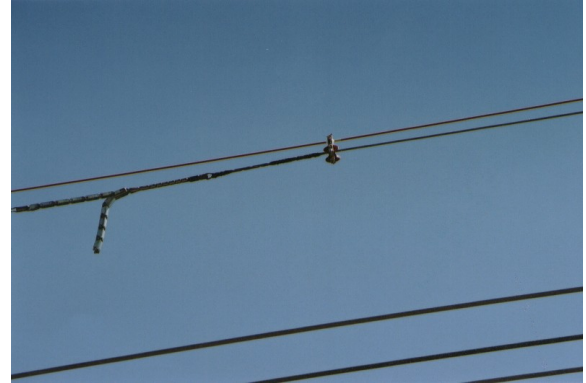
Fig. 4 - Counterweight Tail Device
